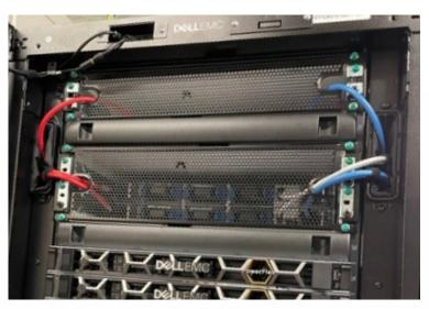
2 or 3 RU Ducts allow for switch cold air to be routed to the inlet of the switch. Power cables are routed thru the front to the cabinet to the back along with the vertical pass-throughs.
