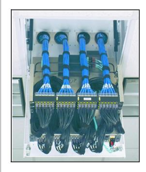
Shown to the right is the recommended patch cord routing from (2) 48- port switches to (2) 48-port patch panels.
