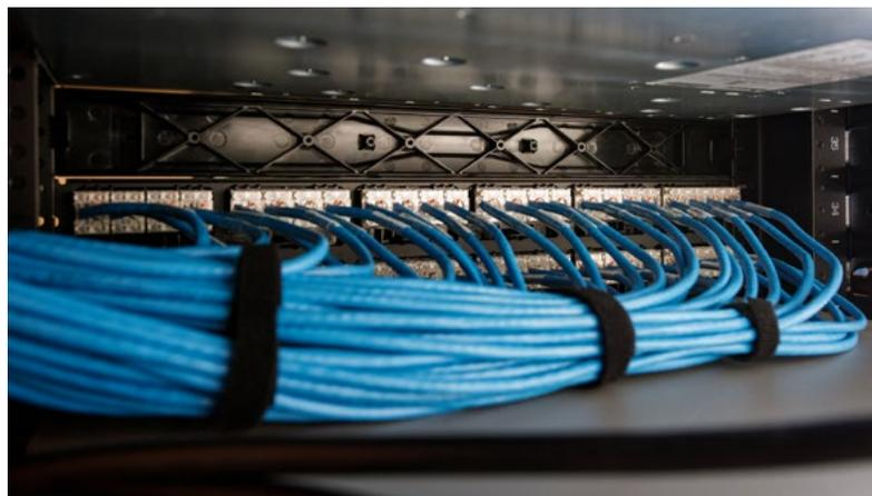
was connected to each switch. The team disconnected each patch cable from the switchport, traced them to the patch panel, and swapped in an appropriately colored cable according to the color-coding method for the associated VLAN. They populated the patch panel jacks one at a time using the color-coding method for the associated VLAN, then reconnected each cord and documented the connection.
