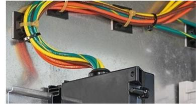
8. Route Sensor Leads and AVT System Cable to avoid sharp edges, pinch points and prevent mechanical damage.
