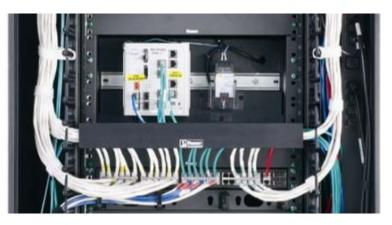
Figure 5. Manufacturing Switch Mounted on a DIN Rail Bracket
