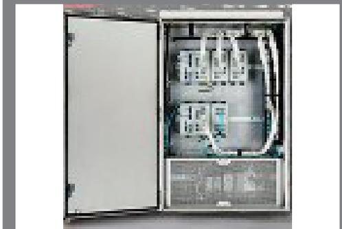
The Panduit Integrated Network Zone System enables network communications between the control room and manufacturing floor within an industrial facility. Integrated with an Allen-Bradley Stratix switch, the pre-engineered, tested and validated system reduces deployment time up to 75%.
