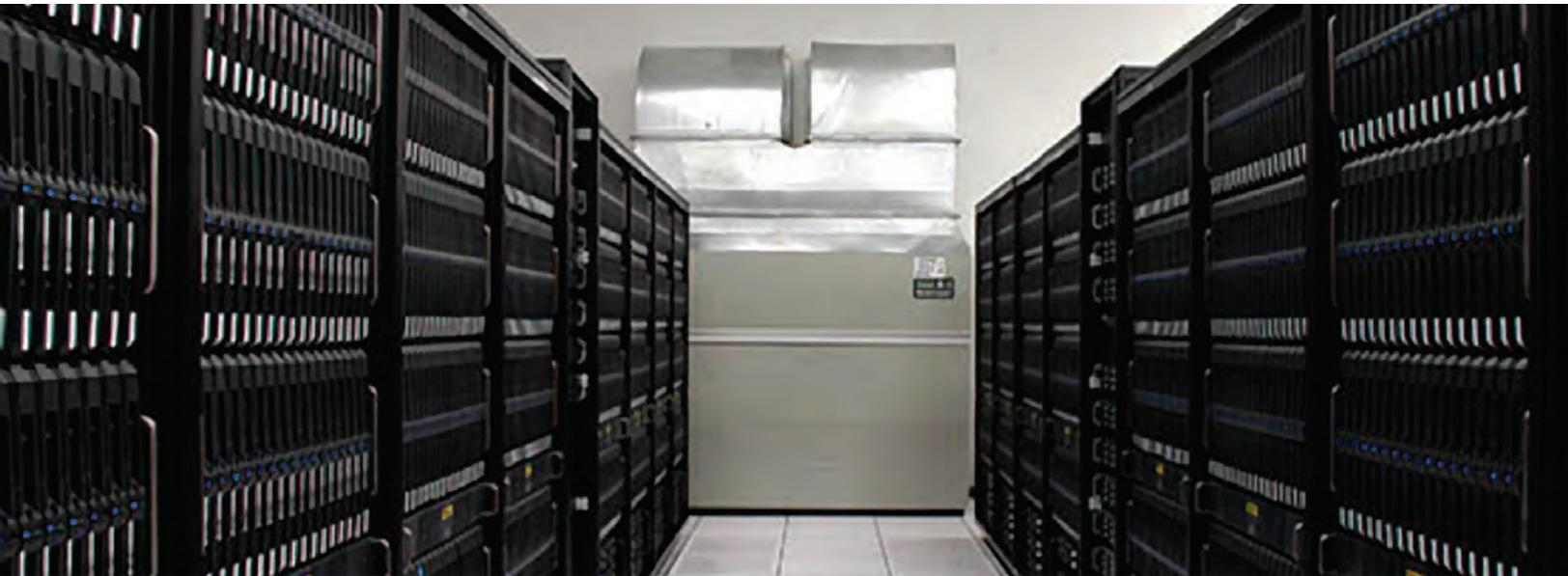
After conducting a careful and thoughtful assessment of the data center, the Panduit team first turned on the two Stulz units which had not been in use. This helped prevent air leaks in the sub-floor and caused the other units to run at a slower rate. Then they installed and ran all of the 13 chilled water cooling units with the Active Control™ feature and replaced 63 perforated tiles with solid floor tiles, which allowed them to raise the sub-floor pressure and lower the fan speeds.
