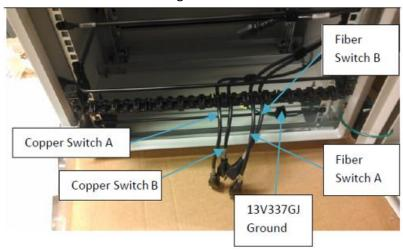
Figure 11: Route the Power Cords into the lower Strain Relief Bracket.
