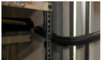
Figure 15: Loom tubing routed around hinge point and rail.
