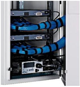
Figure 13: Copper-A (lower) and Copper-B (upper) copper cable bundles attached to strain relief bars.
