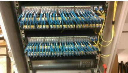
Figure 20: Switch-A (lower) and Switch-B (upper) switches showing fully populated patch cords.
