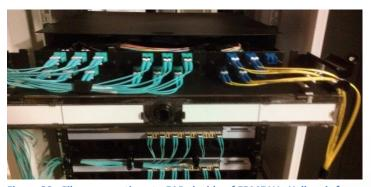
Figure 22: Fiber connections to FAPs inside of FRME1U. Yellow is for management ports. Aqua is for the Fiber Switches.
