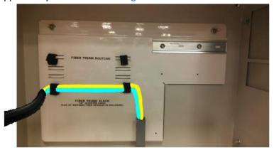
Figure 14: Fiber Trunk routing on Upper Backplane
