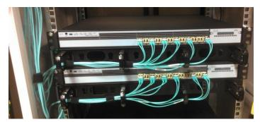
Figure 21: Fiber Switch A and B mounted to front rail showing fiber cable rounting.
