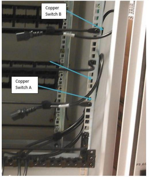
Figure 10: Copper Power Cables A and B. View looking from the rear of the enclosure. Arrows indicate Tak-Ty locations.
