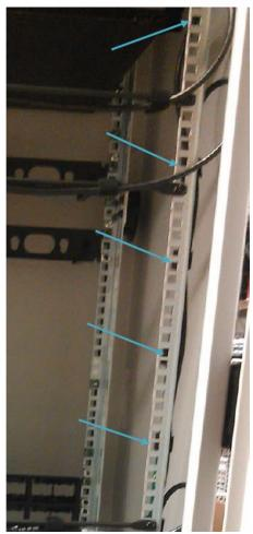
Figure 9: Fiber Power Cables A and B. View looking from the rear of the enclosure. **Arrows indicate Tak-Ty locations.**
