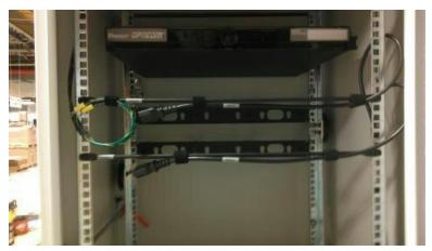
Figure 24: Horizontal support bar with ground cables and AC power cords.
