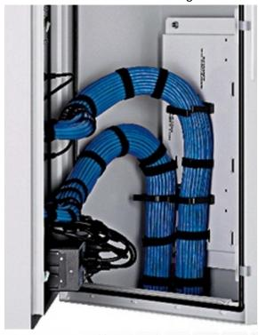
Figure 12: Copper Cable Routing showing Copper-A on the left and Copper-B cables on the right.
