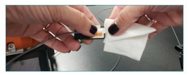
Figure 8: Example method of cleaning the bare fiber(s).
