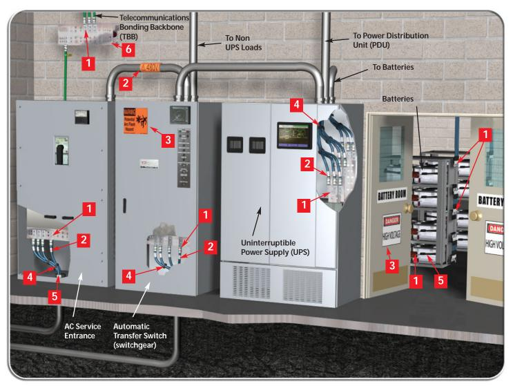
The automatic transfer switch (switchgear) is connected to the utility and generator sources, and is routed to the uninterruptible power supply (UPS). The UPS includes backup batteries and supplies power to the electrical distribution system which allows time for the backup generator to start.
