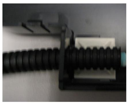
3. Secure corrugated tube and cable loosely to the anchor installed in Step 1 using small Pan-Ty. The fiber cable should be able to be pulled through for terminating the fiber ends.
