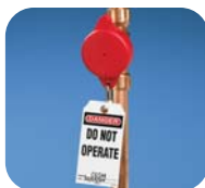
Gate Valve Lockout
