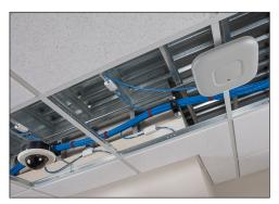
In today's enterprise, things are looking up ... literally. Look into that air-handling space above the ceiling tiles and you're likely to find wireless access points, security cameras, and connections for audio-video equipment, safety systems, and more.
