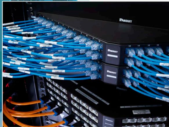
Cables with smaller diameters as well as angled connectors help address these issues. For example, 28AWG patch cords are smaller in diameter and require half the space of standard patch cords. They increase port number visibility, and create more space for plug access, more clearance to route cords, and allow new configurations for more effective use of high-density panels while aiding airflow and cooling.
