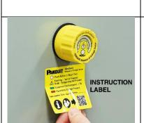
Install Instruction Label directly under or next to the Indicator Module on the exterior of the enclosure (see Note 1). Mark the label to indicate where in the circuit the AVT is installed.
