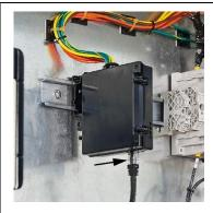
Insert the other end of the AVT System Cable in the connector on the bottom of the Isolation Module.
