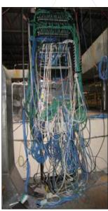
Figure 2. Poor Industrial Network Installation Can Generate Unacceptable Downtime Risks
