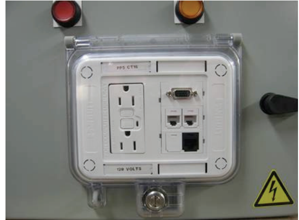
Figure 4.8-5. Data Access Ports manage risk in industrial settings by providing access to the network without opening the control panel.
