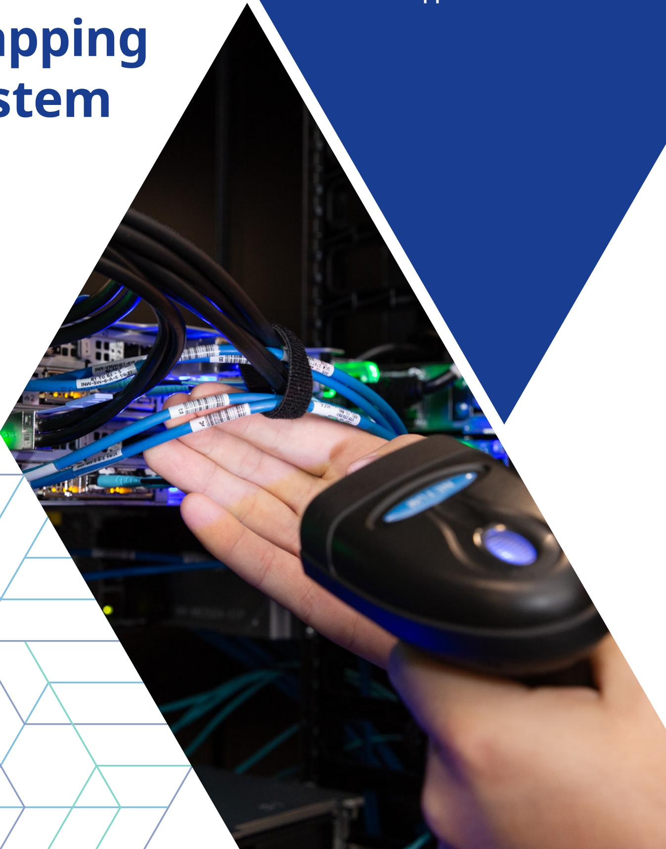
The *RapidID*™ Network Mapping System automates labor-intensive and error-prone cable documentation, resulting in a faster, easier way to place and trace cables and patch cords. It is a practical alternative to traditional manual approaches that are ideally suited for building a new telecom room, locating installed cabling, or replacing a network switch.
