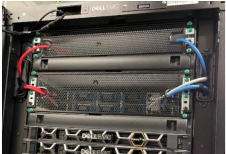
2 or 3 RU Ducts allow for switch cold air to be routed to the inlet of the switch.
