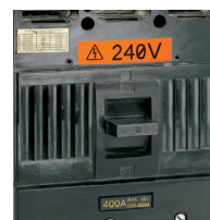
Electrical Hazard Labels
