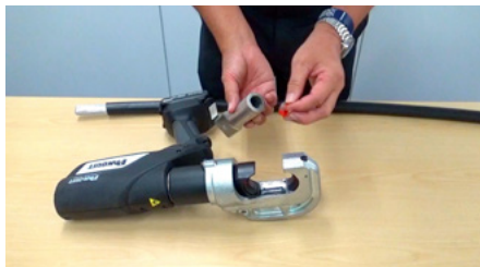
4. The inside of the aluminum terminal contains a compound.
